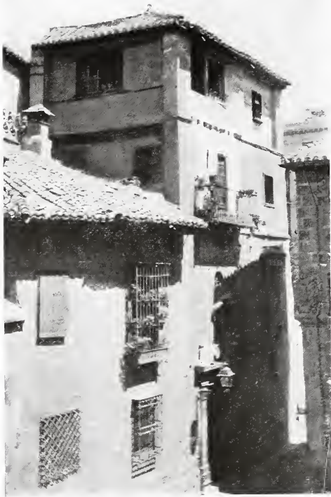
Granada Grilles and Balconies.
